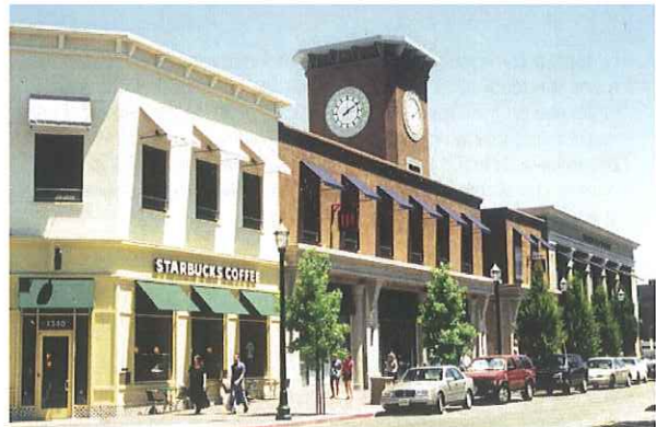
Structured parking is provided on the second and third floors of this Walnut Creek commercial development.
