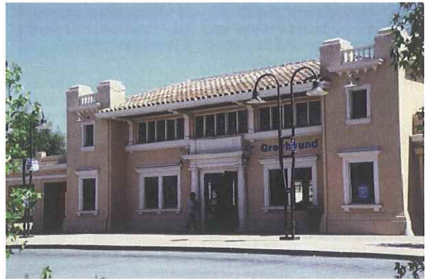
Built-up cornices, sills, and other ornamental features should be used to add pedestrian scale and interest to simple wall surfaces.
