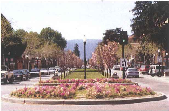
This broad median in Downtown Mountain View creates an attractive, memorable streetscape. It is similar in width to the recommended design for Main Street.
