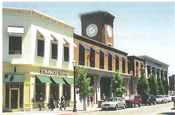
Recent development in Walnut Creek is shaped to create a pedestrian oriented commercial district.
