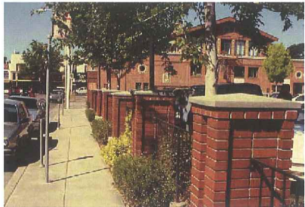
This combination of brick piers and open fencing complements the principal building and screens the adjacent parking lot.
