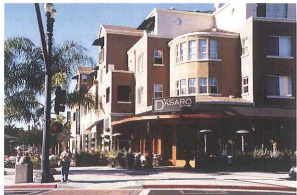
Building entrances shall be located on the front building façade or a fronting building corner.
