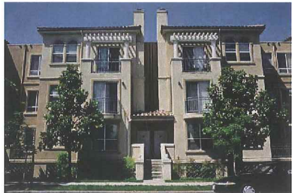
Multi-unit residential buildings should be designed to express individual units within them.
