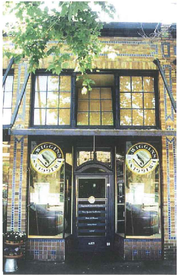
This storefront entrance is highlighted by a canopy, transom windows, and recessed doorway.
