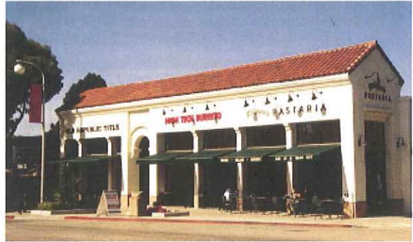
Highlighting building bays with pilasters adds interest to a simple building form.
